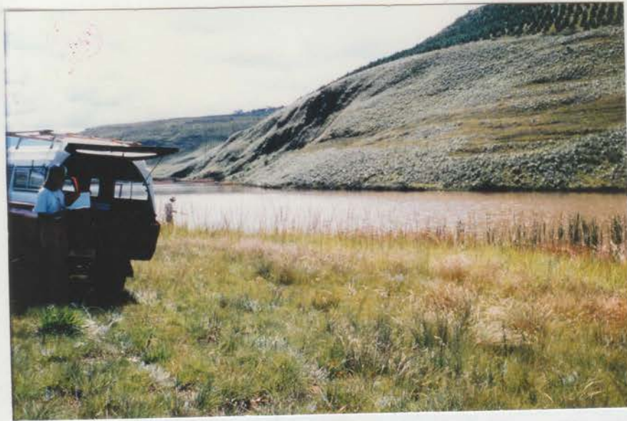
Plate 25. Site 39. Maclear Municipal Dam on tributary of Mooi River.
