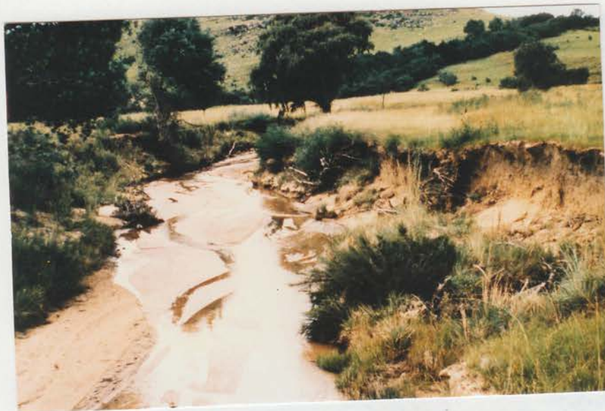
Plate 42. Site 29. Tributary of Nqancule River at Two Streams. Banks eroded and stream heavily silted.
