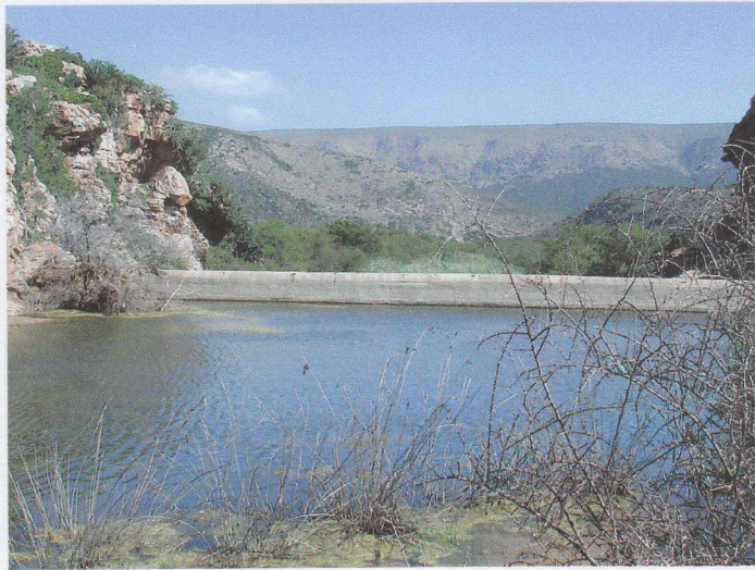
Figure 18. Existing dam wall across Kabouga River, upstream of proposed dam.
