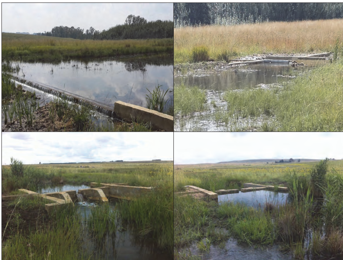
Figure 4.2 The concrete structures that were built to regulate flow during the rehabilitation of the wetland
