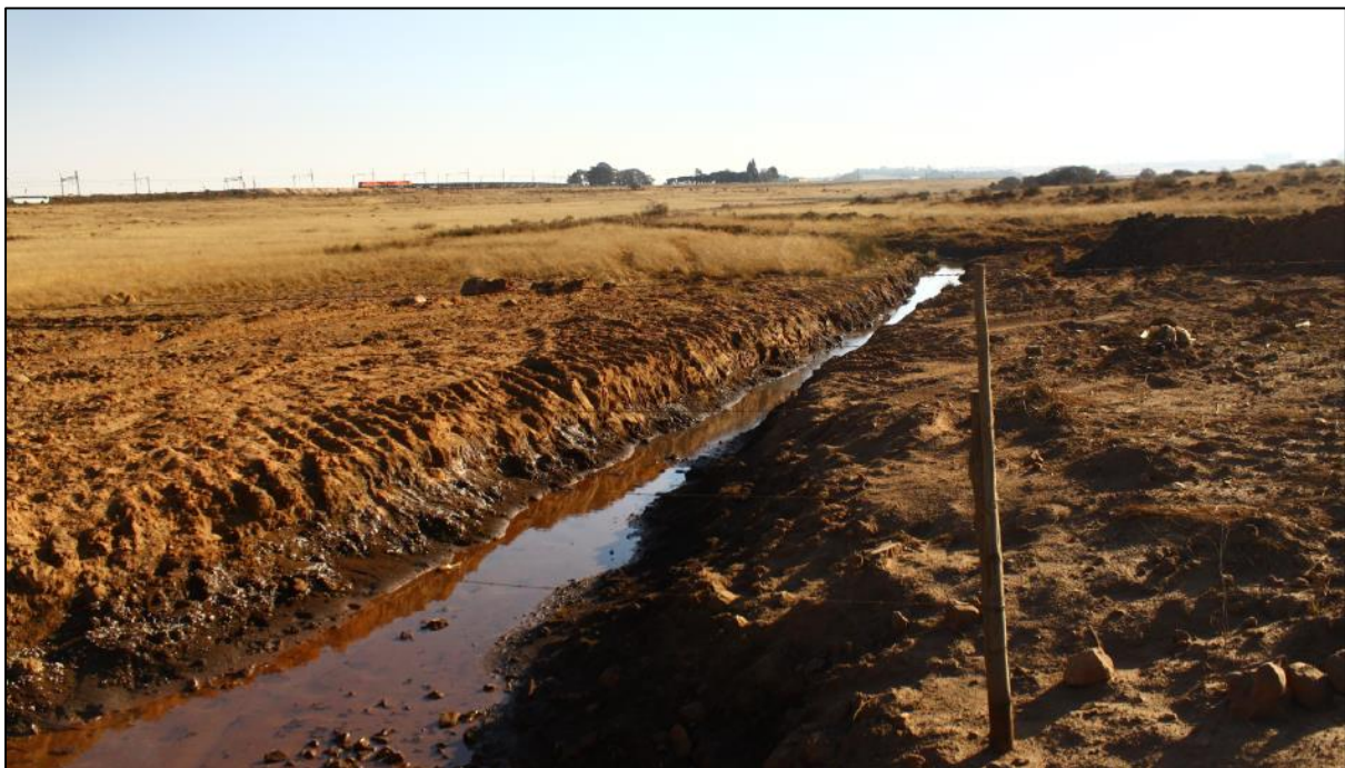
Figure 9: Blesbok River at Vlak5 cleared of sediment build-up with recreation of channel
