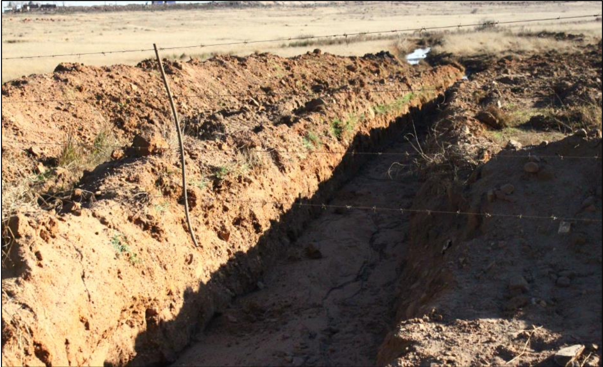
Figure 10: Side channel with steep banks catering for stormwater runoff at Vlak5
