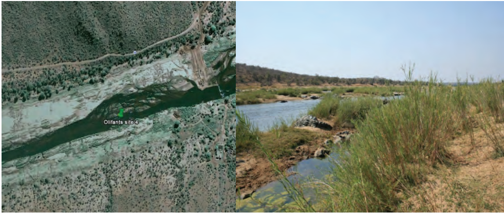
Figure 11. Site 4 situated before the confluence of the Olifants and Letaba Rivers (Google Earth).
