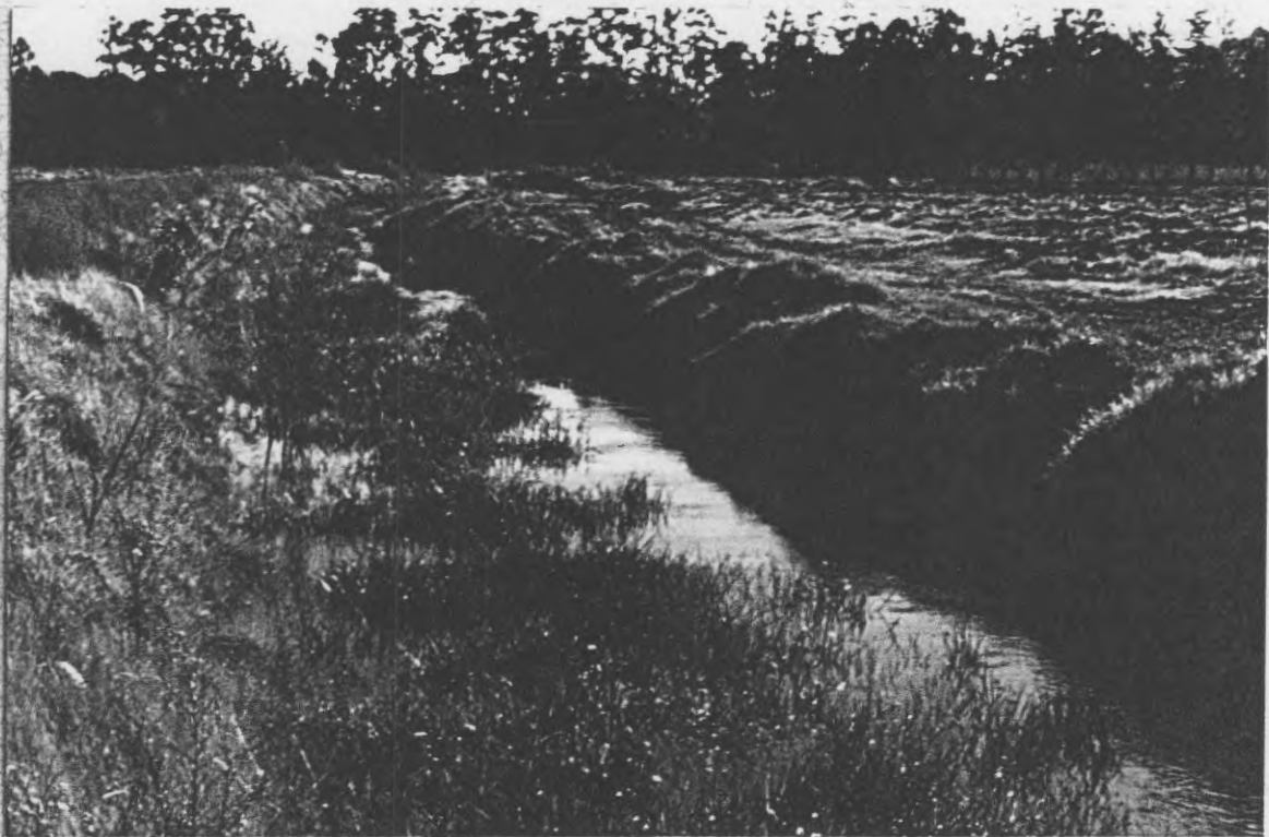
Plate 6. A canal with established bank vegetation is less susceptible to erosion.
