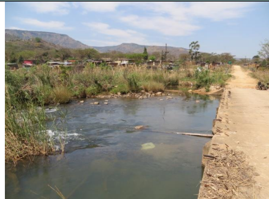
Figure : Downstream view of the Eland-Linde site (19 September 2012, H.Marais).
