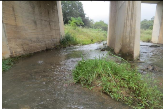
Figure : Upstream view of the Queens River site (27 March 2012, H.Marais).
