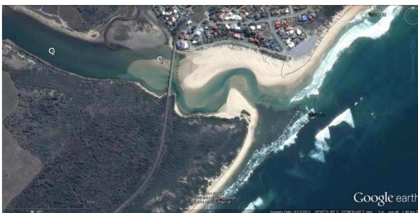
Figure B.1 Accumulation of sediment downstream of railway bridge in the Klein Brak Estuary (Source Google Earth)
