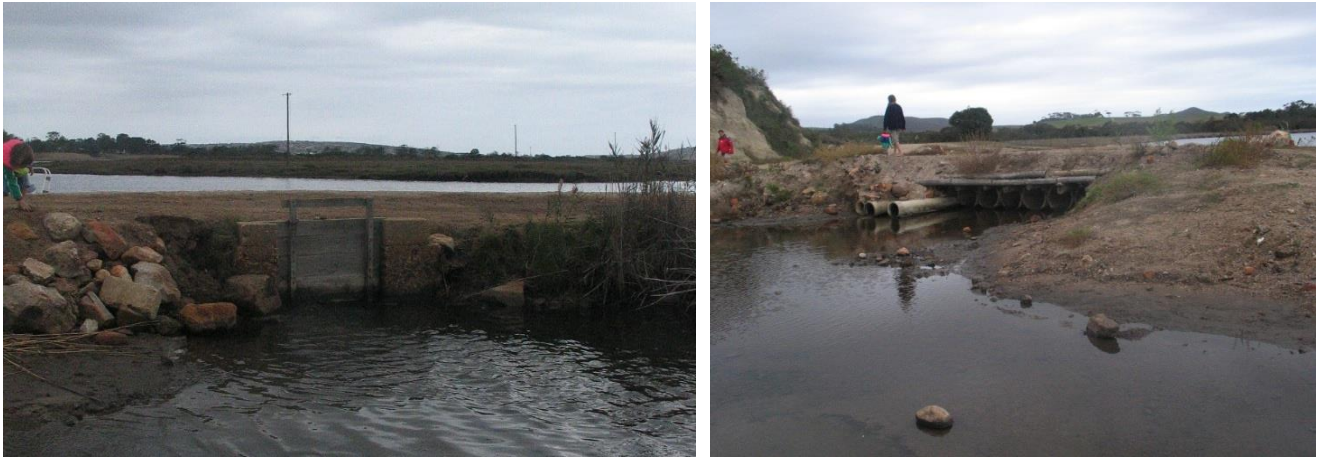
Figure A.7 Roads and blocked culverts preventing tidal flows and salinity penetration into the upper reaches of the Klein Brak Estuary
